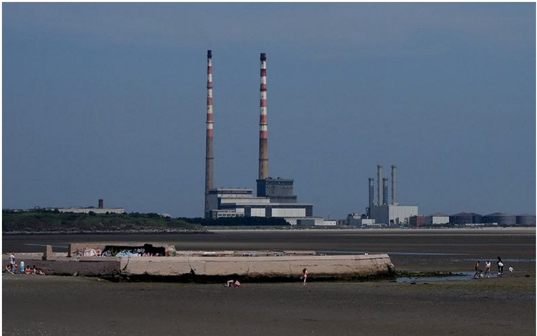
Dublin's Poolbeg Power Station, the two 200m high chimneys even featured in a well known U2 video
